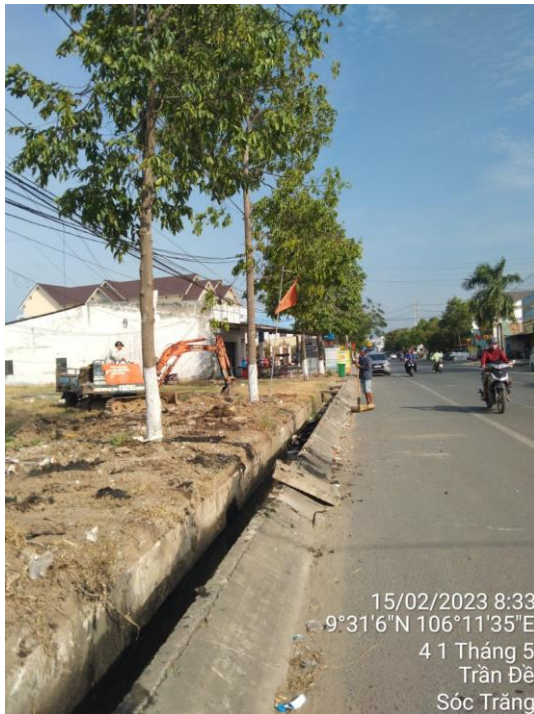
Image of drain clean-up
