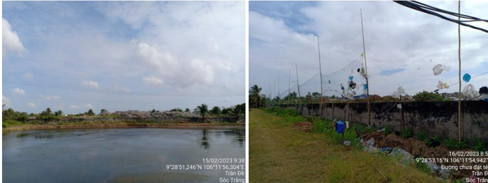
Images of Fencing at the Trung Binh dumpsite
